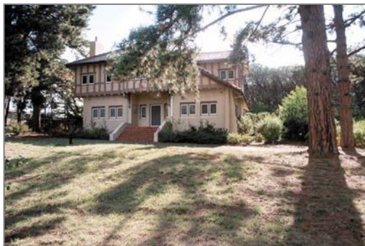
Figure 63: Westridge House from Banks Street and the entrance driveway 2010.
