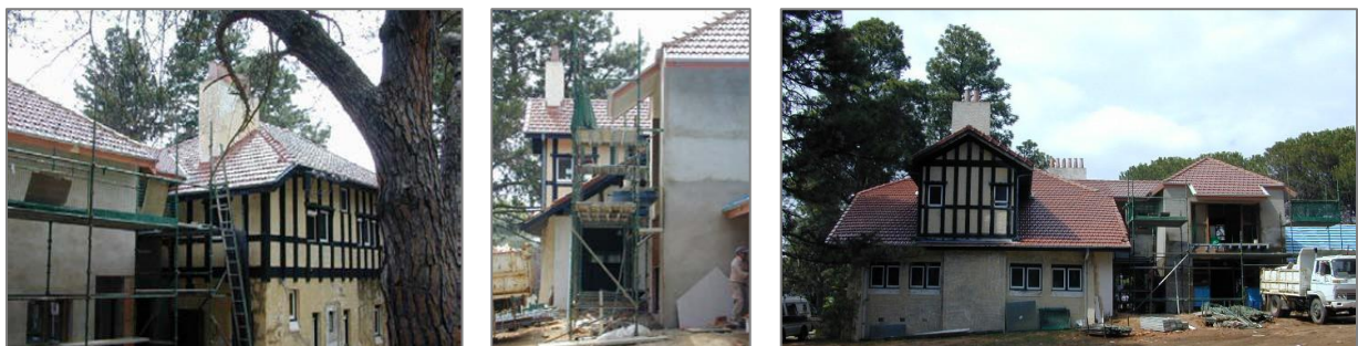
Figure 49: 2001 and 2002 photographs of the extension works
